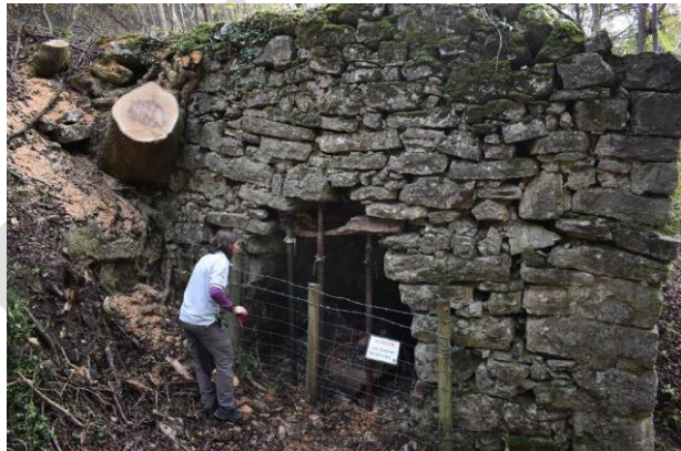
Old limekiln Bat survey by Enfys Ecology before repair work begins →
